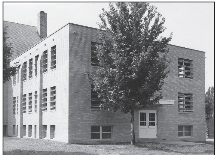
The Annex was built onto the northwest corner of the sanctuary in 1958.
